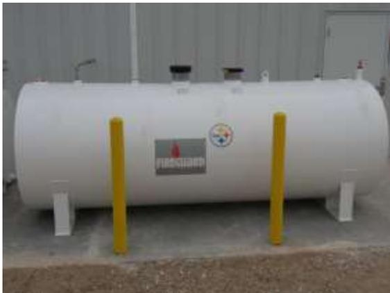
A UL2085 **Fireguard tank** is a tank registered with the Steel Tank Institute and only available from a STI member. The Fireguard tank is a double wall tank that contains insulation between the inner and outer tank protecting the product from ambient temperature variations and exceeds the UL 2-hour fire test.
