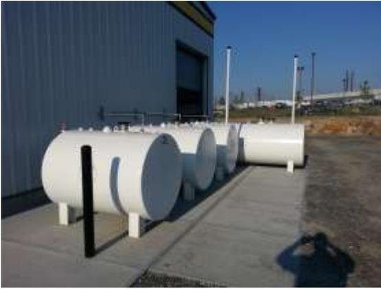
This was an installation of mixed tanks, a 1000 gallon Flameshield for clean gas, a 500 gallon Flameshield for dirty gas and two 500 gallon UL142 tanks for oil & coolant.
