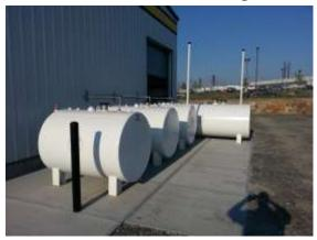
This was an installation of mixed tanks, a 1000 gallon Flameshield for clean gas, a 500 gallon Flameshield for dirty gas and two 500 gallon UL142 tanks for oil & coolant.
